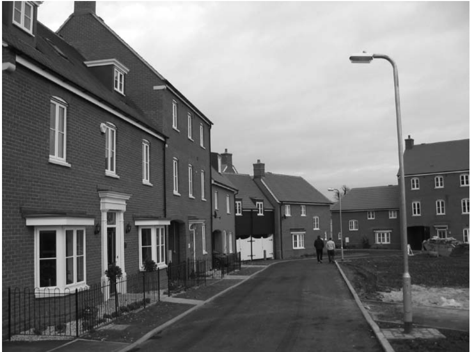
Figure 4.5 The BAe site development approaching completion. Architecture is by Reeves Bailey. Note the provision of small front gardens. See also Plate 4.2. Source: Chelmsford Borough Council.
