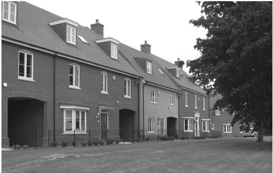
Figure 4.6 The completed BAe site development showing frontage to the local open space. Source: Chelmsford Borough Council.
